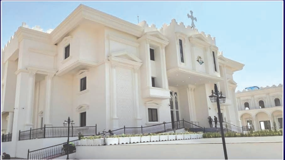
New Patriarchal Headquarters of the Assyrian Church of the East in Erbil, Iraq
